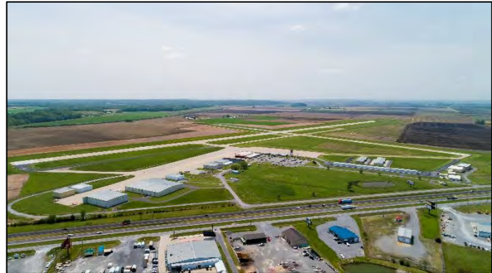
Figure 47: Cape Girardeau (CGI) Regional Airport
