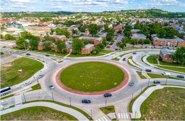
Roundabout on KY 9 in Campbell County
